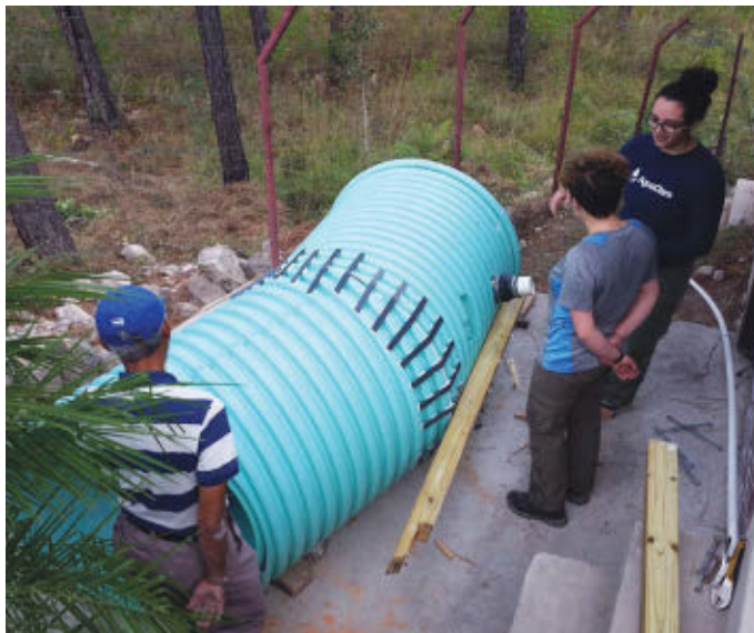
AguaClara team leads Zoe Maisel '18, center, and Erica Marroquin '18, right, are pictured with Jorge Dueñas Carcamo of Agua Para el Pueblo, in Cuatro Comunidades, Honduras. The three were preparing to install AguaClara's first 1 liter-per-second system.
